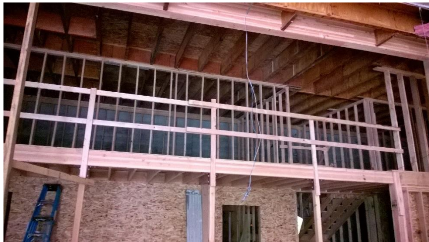
Level 2 class rooms on West end
